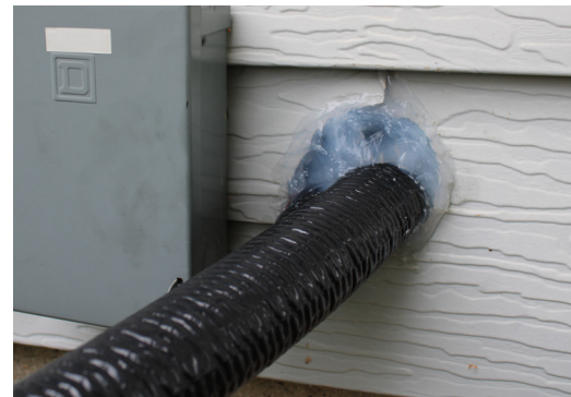
Be sure to air seal all wall penetrations.
