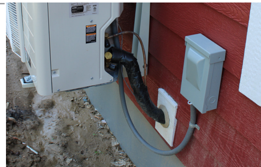
Ensure that the insulation is thorough and covers the entire line set, as shown here.
