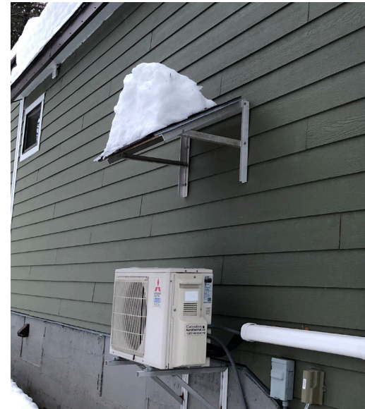
Proper outdoor placement, showcasing a drip cap/snow shield.
